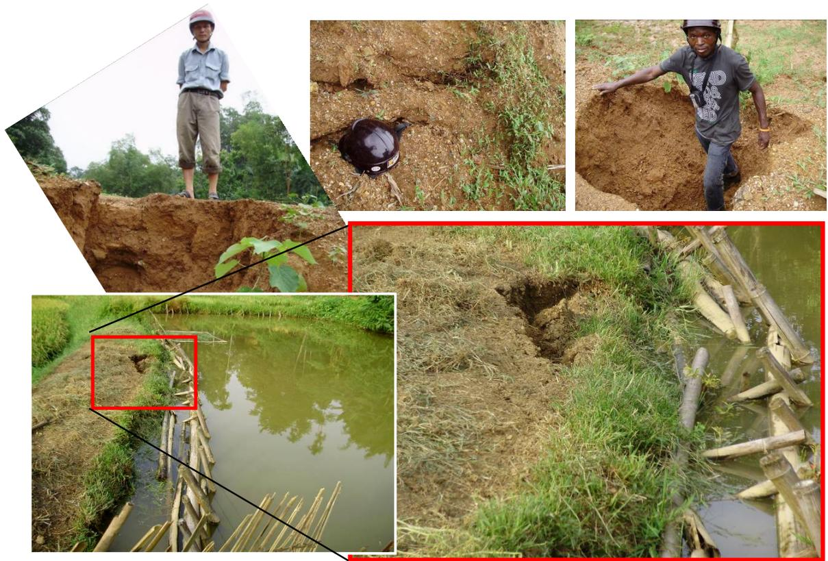
Figure 3.7: Cracks on dikes and ponds
