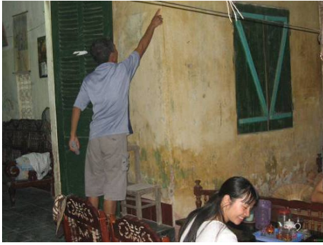
Indication of flood water level
