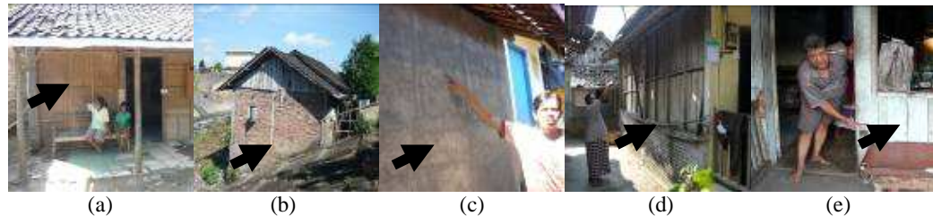
Figure 6-3. The types of wall (a) bamboo (b) brick (c) concrete (d) mixed (e) wood
