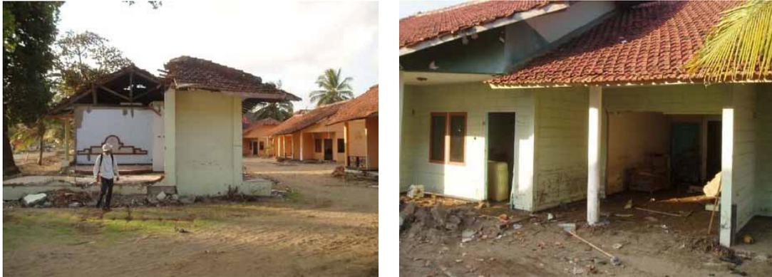
Figure 5-17. In a flow depth of about 2 m, the buildings in the first row toward the sea were heavily damaged (left) while those in the third row had suffered little structural damage (right) (Reese *et al.*, 2007)
