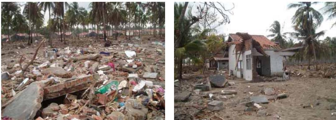
Figure 5-13. Most of the traditional brick construction type collapsed after inundation of 3 meters (left). There were a few partially intact (right) (Reese *et al.*, 2007)
