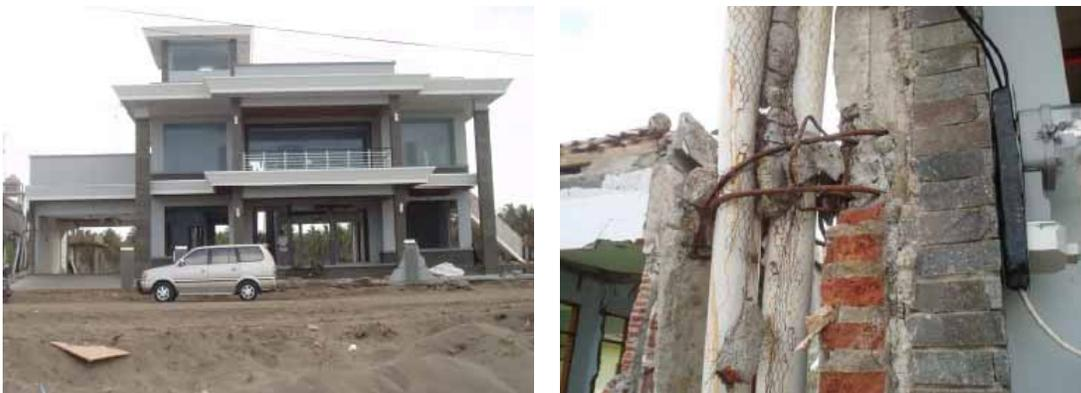
Figure 5-15. Damages on a well engineered *RC-frame with brick infill walls* building after inundation to a depth of 3.8 meters (left) and the detail of the reinforcement (right) (Reese *et al.*, 2007)
