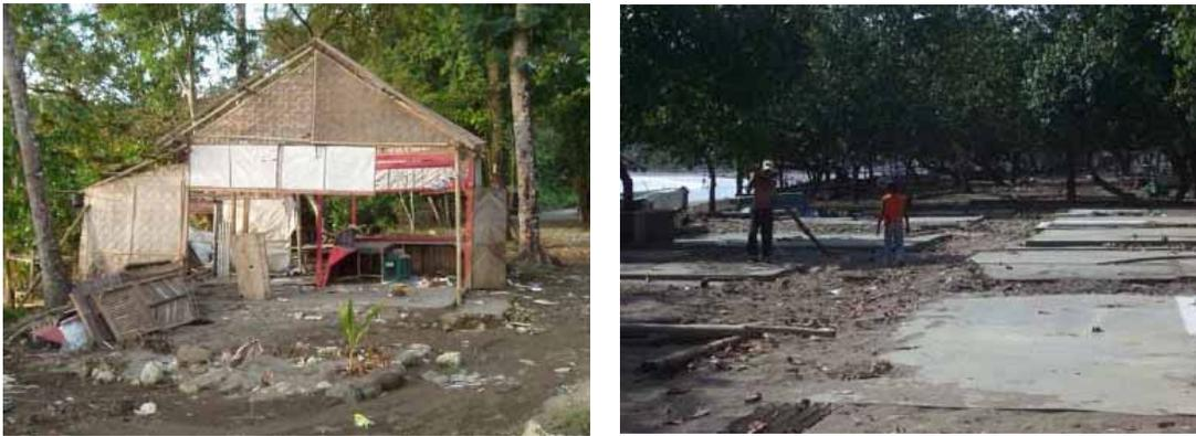
Figure 5-12. Damage to timber/ bamboo construction type after inundation to nearly 1 meter depth (left) and 3 meters depth (right) (Reese *et al.*, 2007)
