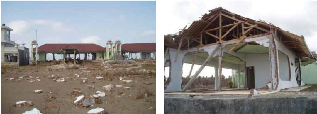
Figure 5-14. Debris field inland of the damaged buildings (left) the damage of *traditional brick with RC-columns* to a flow depth of 3.8 meters (right) (Reese *et al.*, 2007)
