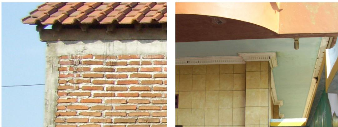
Figure 6-12. 10 cm x 10 cm to 20 cm x 20 cm column dimension for *traditional brick with RC-column* construction type (left) and at least 20 cm x 20 cm column dimension for *RC-frame with brick infill wall* (right) (fieldwork doc.)
