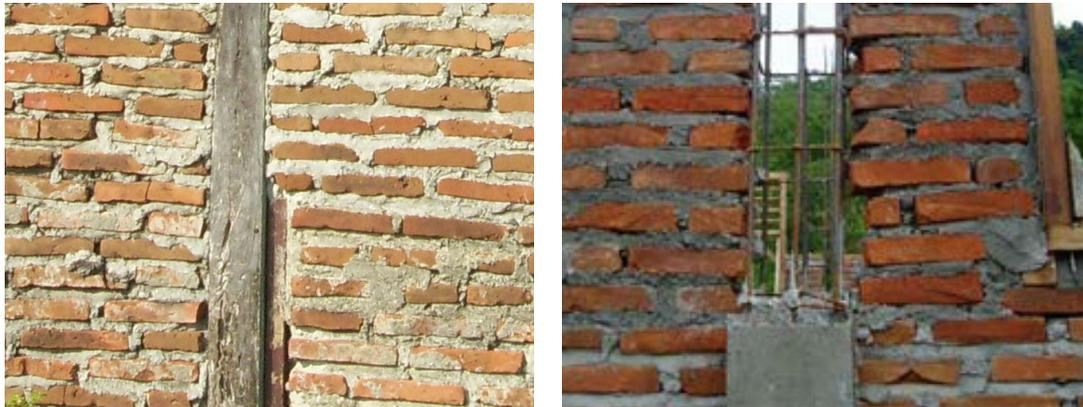
Figure 6-11. *Traditional brick* construction type (left) and reinforced concrete column added to strengthen the structure and to create a *traditional brick with RC column* (right) (Boen, 2006)
