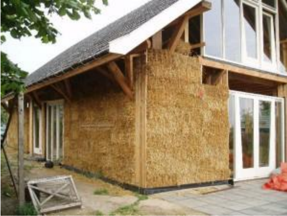
Figure 16 Straw and wood construction
