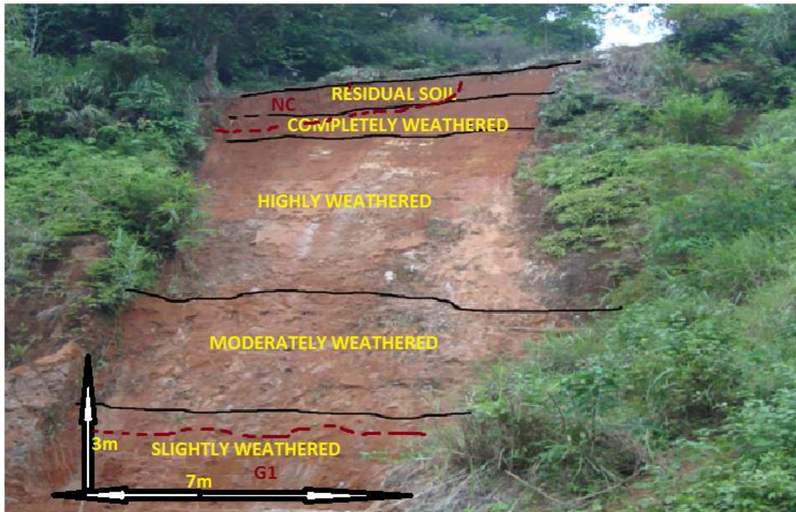
Figure 4.6: The different lithologies and degrees of weathering (see table 3.3) for the recent cut of Slope Y27 (Direction of view - 040°)
