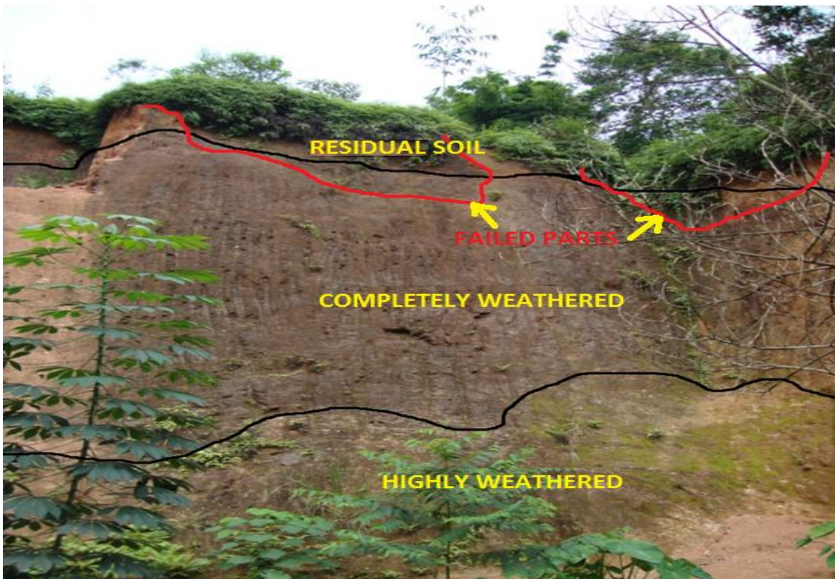
Figure 0.18: The different lithologies and degrees of weathering for the recent cut of Slope Y11 (Direction of view - 330^{\circ} )
