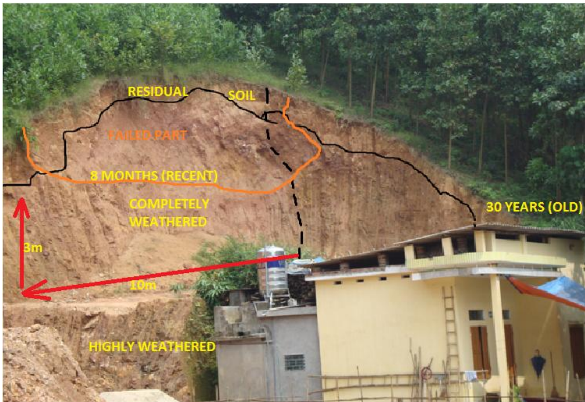
Figure 0.27: The different lithologies and degrees of weathering of Slope Y21 (Direction of view - 020°)
