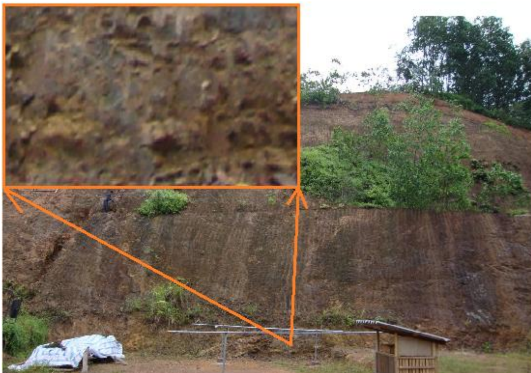
Figure 0.54: Typical slightly weathered rock materials from the research area - (cut slope Y2 – 22/09/2010 – 11.38hrs; scale – 1:8000) (Inset - scale – 1:3500)
