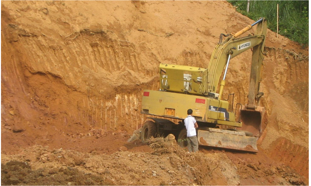
Figure 0.1: A typical excavator machine used for the cutting of slopes in the research area
