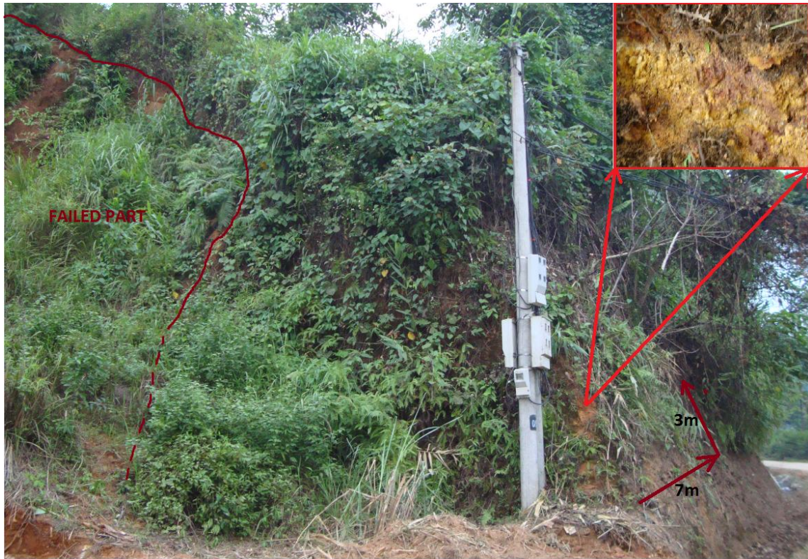
Figure 0.29: The old cut of Slope Y27 (Direction of view - 040°)
