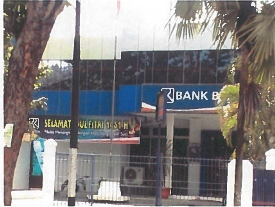
Figure 5-18: the Concrete frame building In Sumuran Sub village
