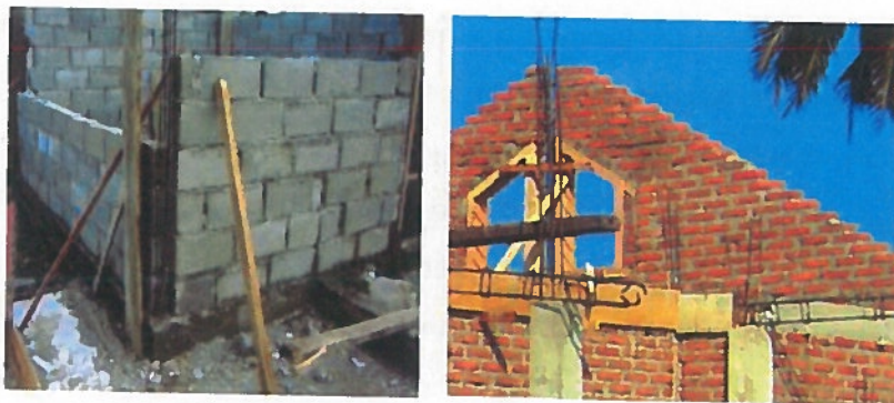
Figure 2-13: Confined masonry construction in Indonesia
