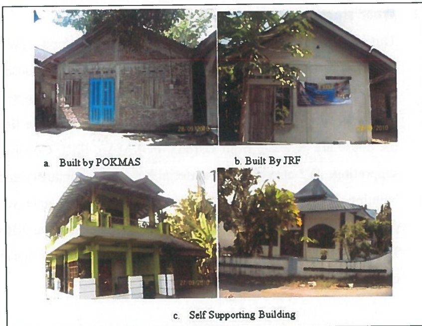
Figure 5-14: Sample of Reinforced Masonry Building structure in Palbapang Village
