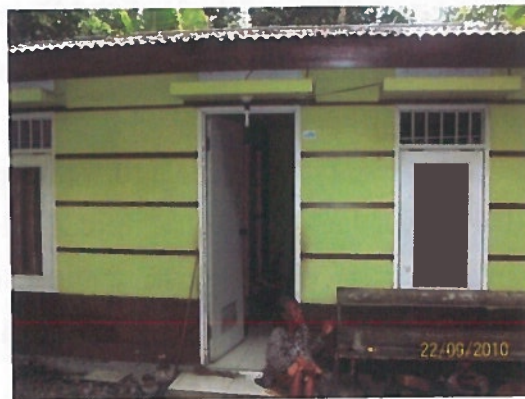
Figure 5-17: The light steel frame building In Karasan Sub village
