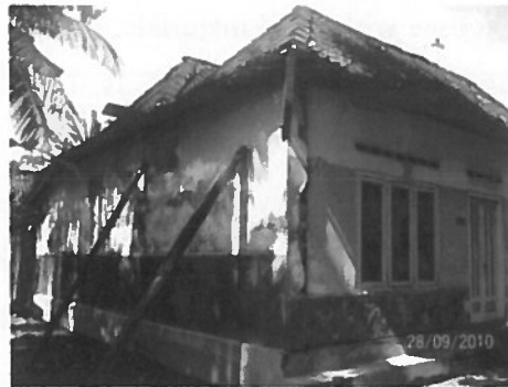
Figure 5-15: Sample of Unreinforced Masonry building in Palbapang village
