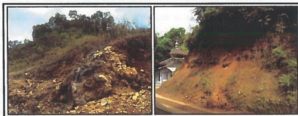
Figure 4.3. Site 8 showed limestone of upper portion of Jonggrangan Formation (left), site 1 showed conglomerate and sandstone of lower portion of Jonggrangan Formation (right).
