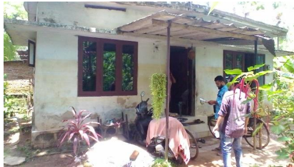
Figure 15 : Flood water mark Pandanad panchayat
