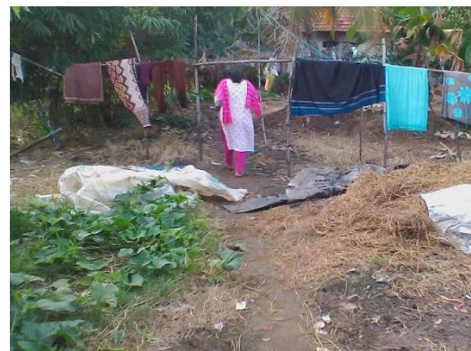
Figure 14: House damaged by landslide in Chittar panchayat
