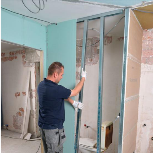
Figure 1 - Metal stud wall system
