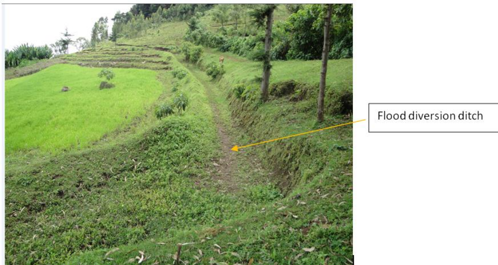
Figure 5-7: Water diversion ditch
