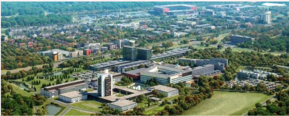
Figure 1, 146-hectare campus of the UT
