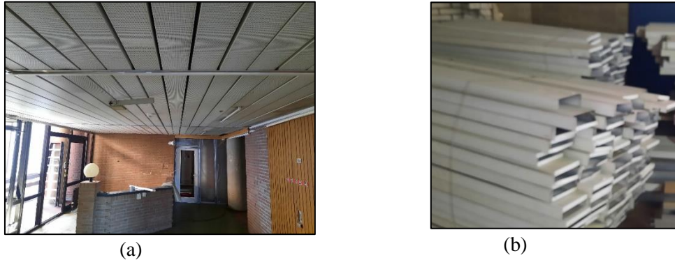
Figure 3 - (a) ceiling panels with asbestos pollution, (b) cleaned ceilings panels stored at project location (Project 2)
