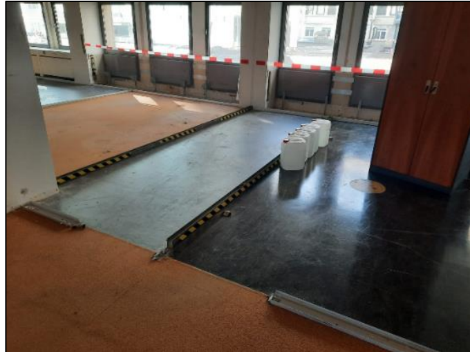
Figure 4 - Rails cannot be disassembled while maintaining quality as it is connected to an asbestos polluted floor (Project 3)
