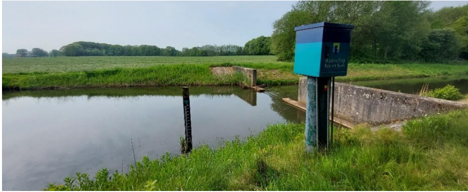
Figure 4: Weir and measurement point 'Overlaat de Kip'
