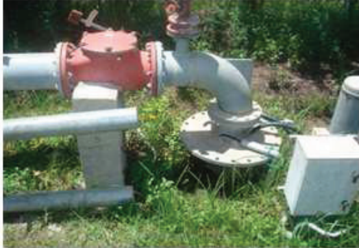
Production well Akaki Wellfield
