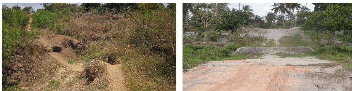
a) Poorly constructed road with no culvert-Mivumoni b) Poorly finished road with a small culvert-Buyuni
