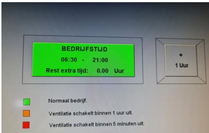
Figure 4-3: Bender panel displaying an OR in daytime operation
