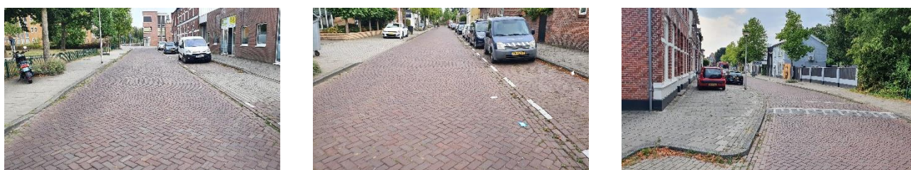
Figure 11: Situation of the Tweede Emmastraat as of September 2022
