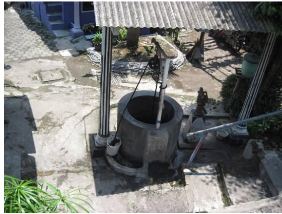
Figure 4.2: Communal well surrounded by impervious surface at Gowongan Village
