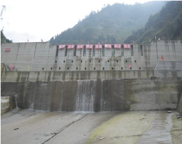
Figure 23 the biggest check-dam in the catchment
