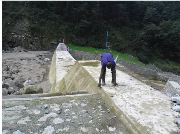
figure24 measuring the width of check-dam (source: fieldwork)
