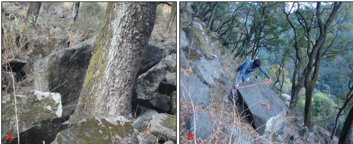
Figure 3-3: (A) A rock stopped by tree and (B) Measurement of fallen block dimension (at Aungi)
