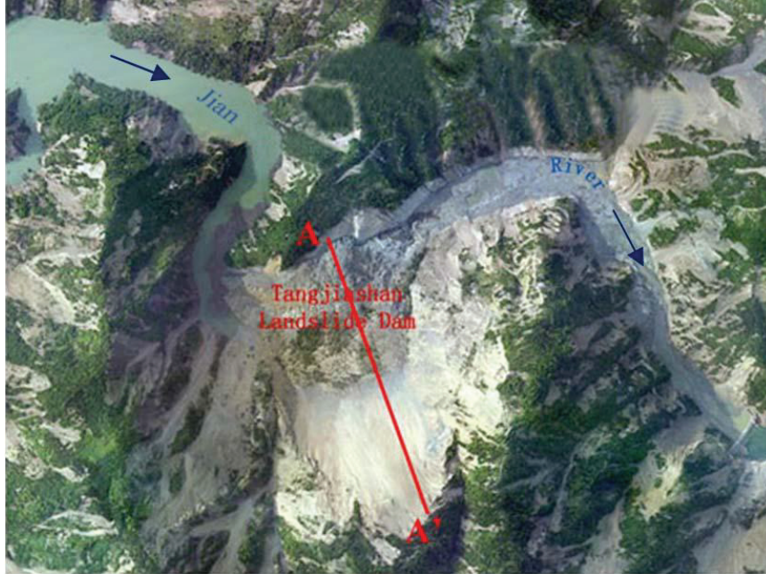
Figure 3-2 Tangjiashan landslide dam blocking Jian River (Cui, et al., 2010); Photo from Ministry of Land and Resources)
