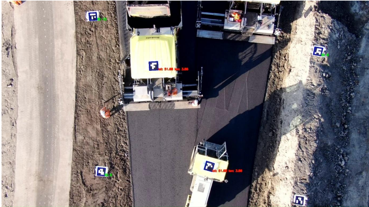
Figure 12: Example of two machineries being detected by the algorithm on OpenCV
