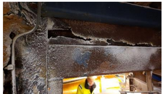
Figure 4 Corrosion damage in the bridge 3 due to salt
