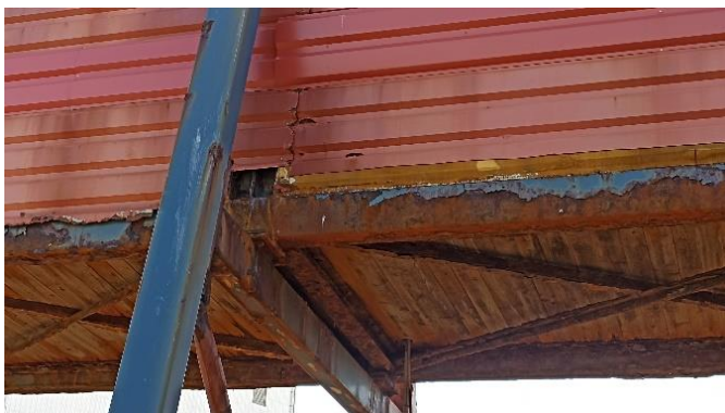
Figure 3 Corrosion damage on the outside of bridge 3
