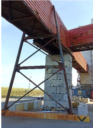
Figure 8 Support Existing bridge in the front with extra concrete support in the back
