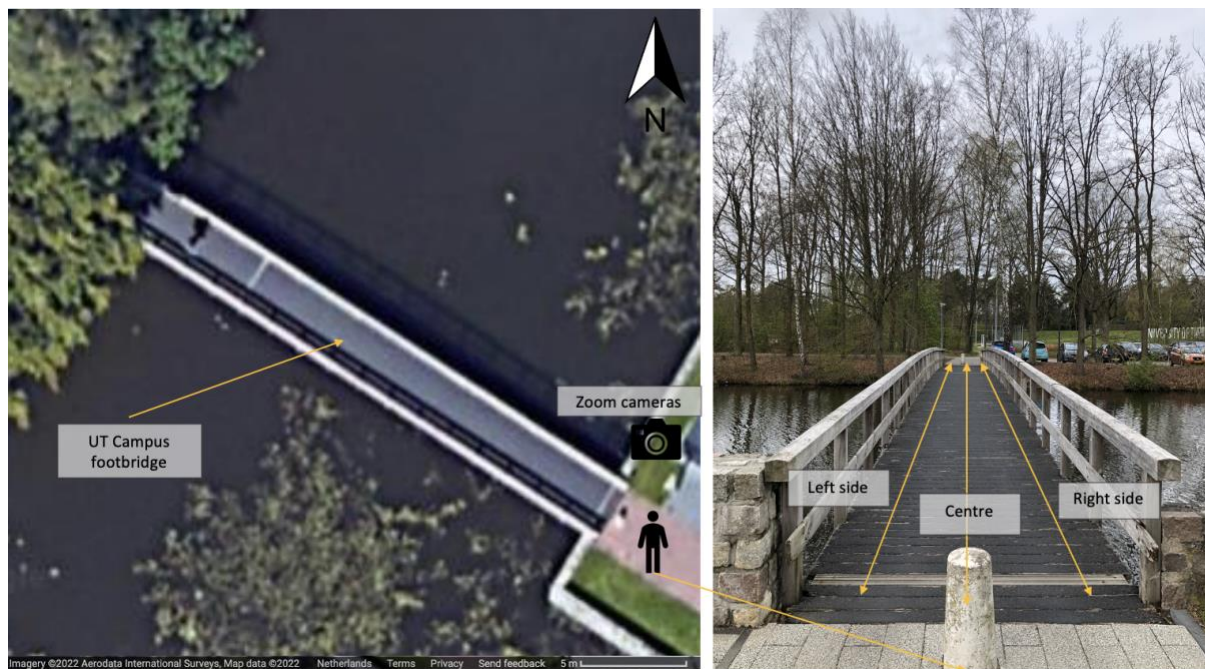
Figure 12 (left) UT Campus footbridge from above and (right) up-close
