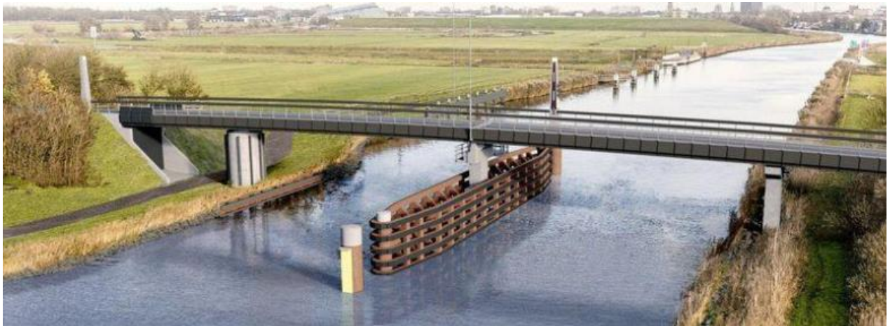
Figure 2: Bio-based bridge (closed)
