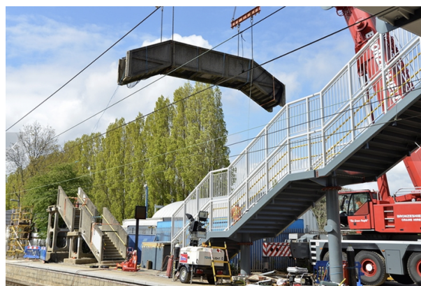
FIGURE 7: Telecrane installing a concrete bridge, (VEDA Associates, 2014)
