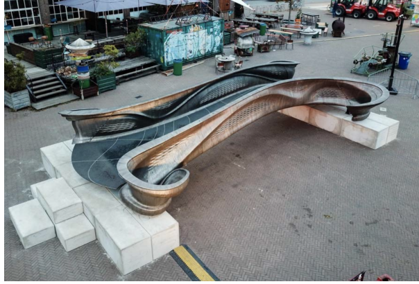
FIGURE 14: Overview of the MX3D metal 3D printed footbridge, (Rolands Kromanis, 2021)
