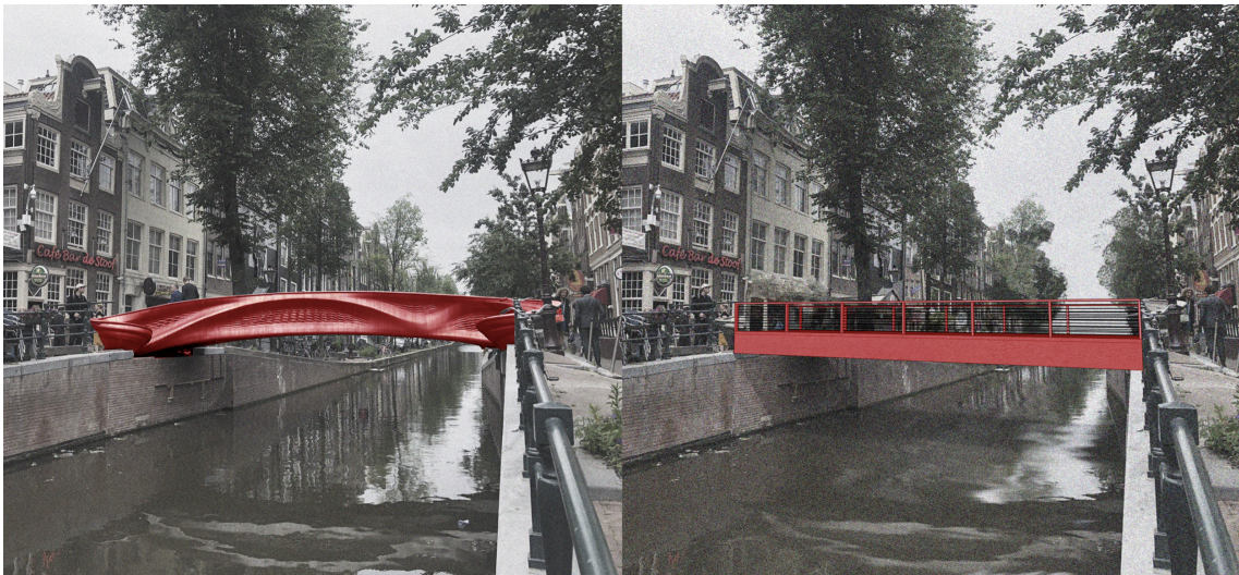
FIGURE 4: Bridges alternatives (3D printed Steel-left and Concrete-right) modeled at the construction location
