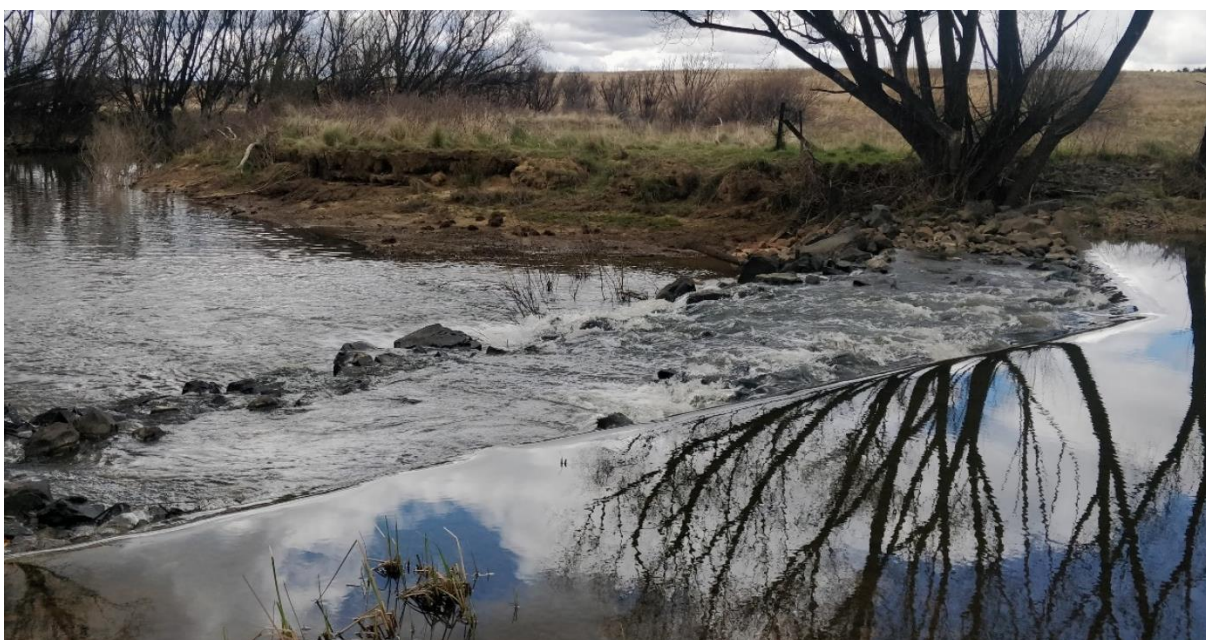
Figure 10 - leaky weir at T2 (own photo)
