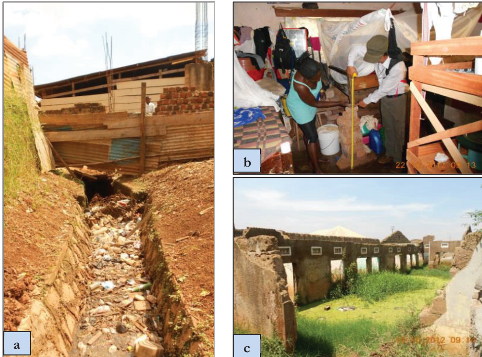
Figure: 1-1 Issues related to flooding (A) House constructed over the drainage channel. (B) Bed raised on stone and belongings hanging on the wall. (C) Abandoned house with stagnant water inside.
