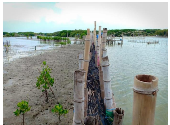
Figure 54, Permeable structure to create favourable conditions for mangrove rehabilitation
