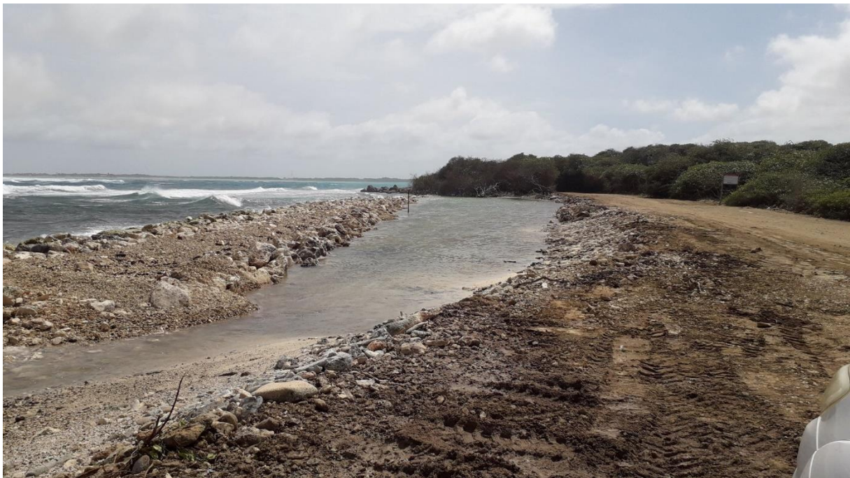
Figure 56, Current situation at Lac Cai were a pile of rocks is deposited perpendicular to the coast in the form of a breakwater
