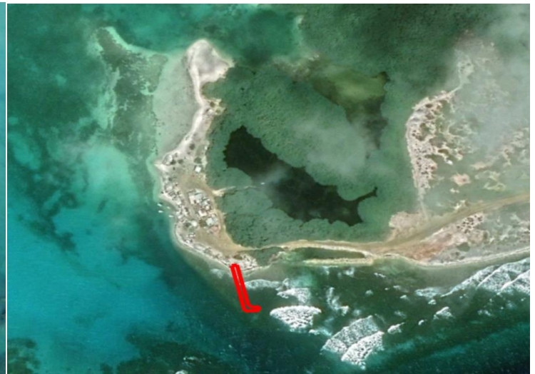
Figure 57, Schematic overview of a groyne at the south side of the beach at Lac Cai (Google Earth)
