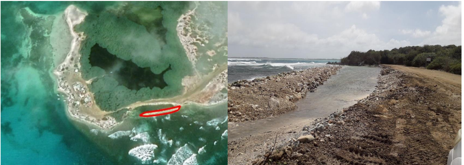
Figure 32, Aerial overview (Google Earth) (left) and photo on sight (right) of the current situation at Lac Cai were a pile of rocks is deposited perpendicular to the coast in the form of a breakwater
