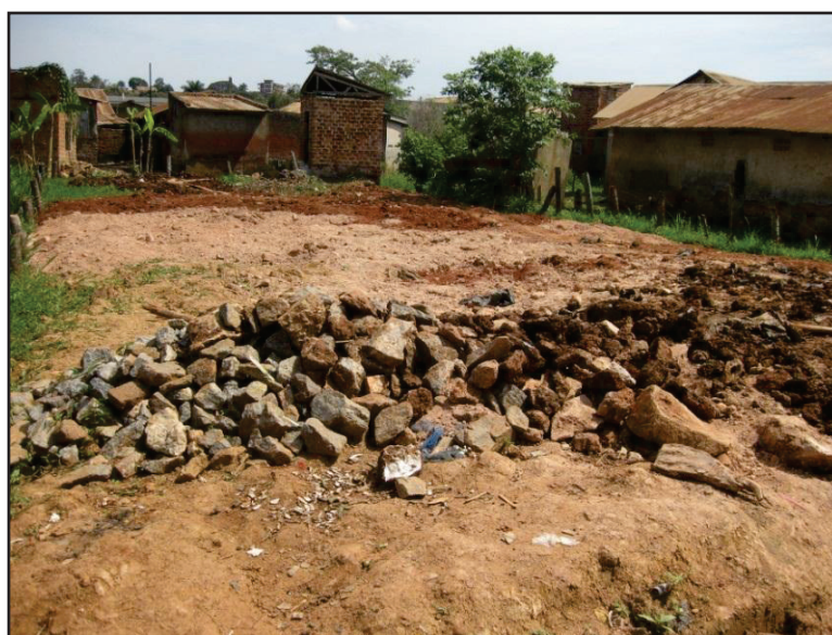
This developer do not care of the effect of sand filling his/her neighbour Figure 4.10: An example of Sand filling by a developer.
