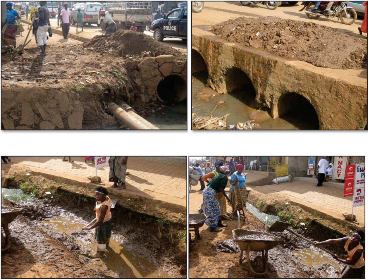
Figure 4.10: Clearing of a drains and water channels as a form of coping strategies the study area
