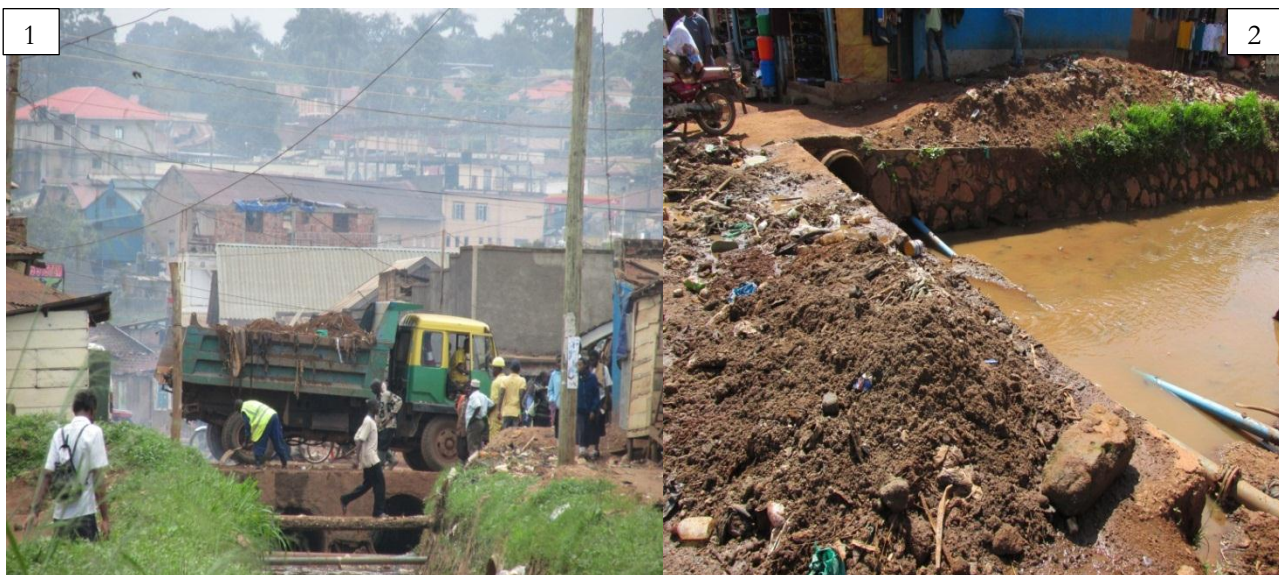
Figure 22: Cleaning of drainage channels
