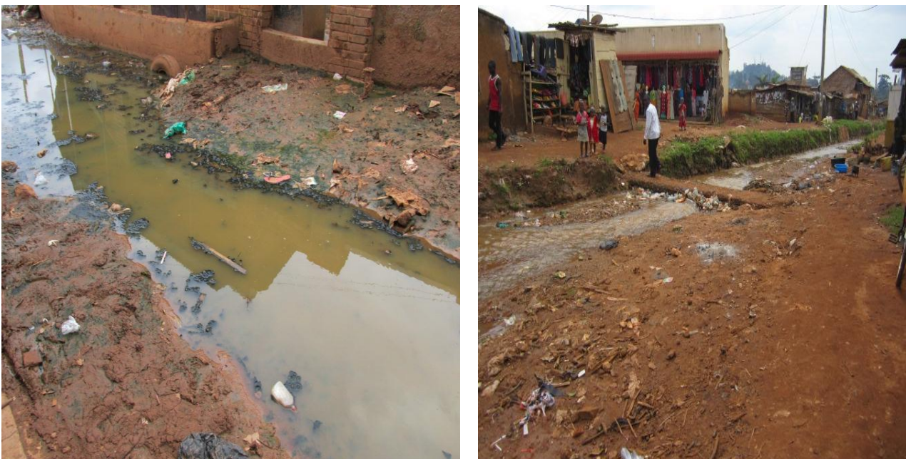
Figure 10: Poorly disposed garbage blocking flow of water in the area.
