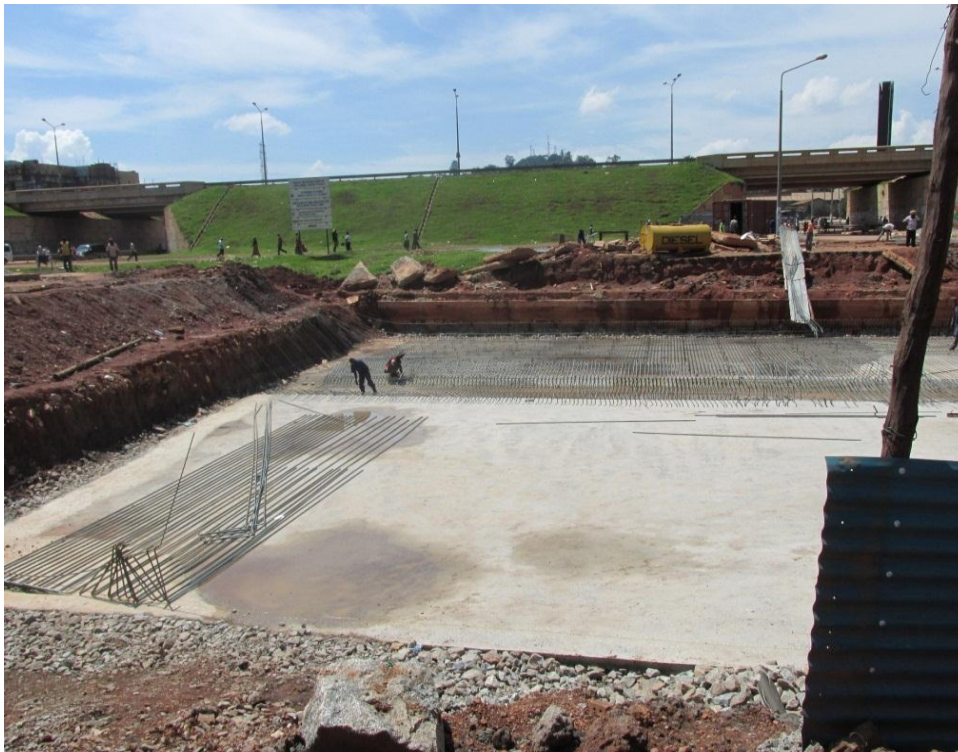
Figure 24: Expansion of Lubigi drainage channel
