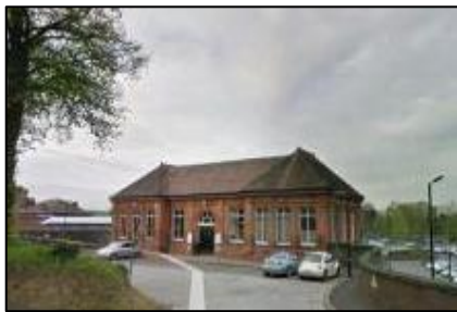
No 1: Central train station building
