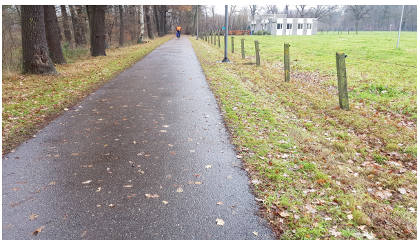
Fig. 2. A two-way isolated bicycle path without markings
