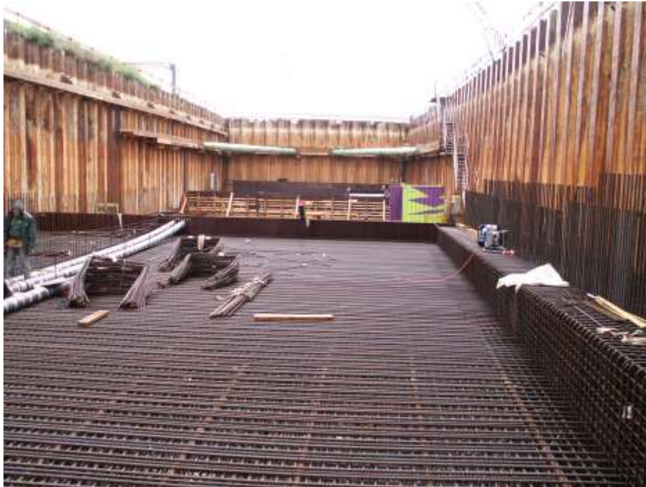
Figure 20-sheet pile used in Galamadammen aqueduct ( (Wiki, 2022)
