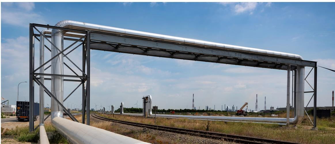
**Figure A.3:** Steam & condensate pipelines crossing a railway with a pipe bridge [8]
