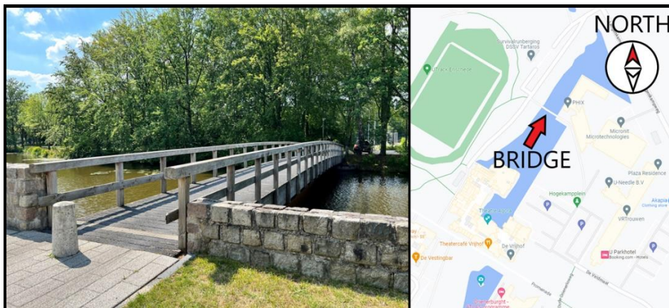
Figure 3: The UT Campus bridge from the East side of HogeKamp (left) and its geolocation (right).
