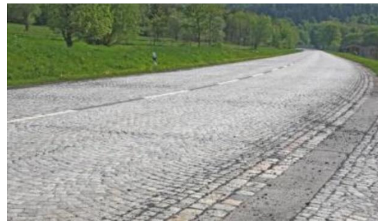
Figure 9: Poor asphalt / good brick paving
