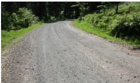
Figure 10: Poor brick paving / compacted rubble
