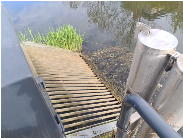
(a) Weir inlet
