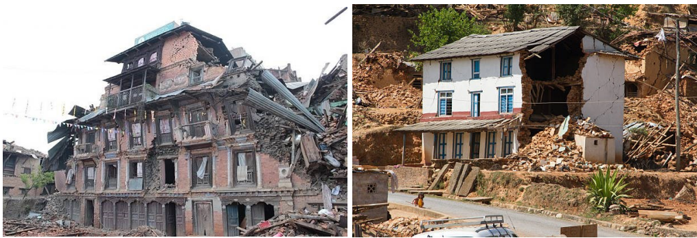
Figure 3.1. Damaged Building Images Samples
