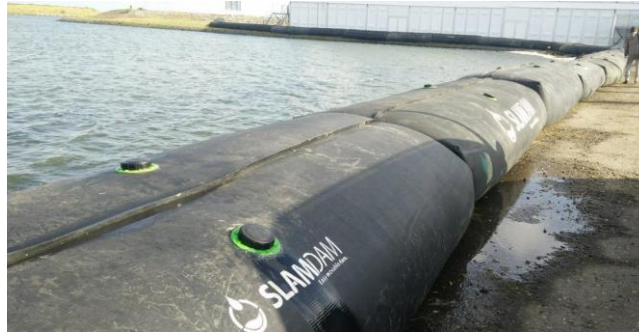
Figure 10: How a water inflatable dam can be used to protect an area from flooding.
