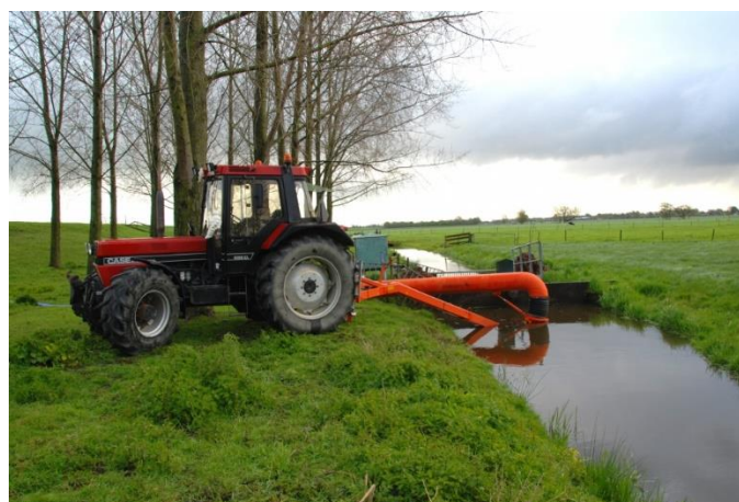
Figure 11: Tractor pump operating for additional pump capacity.
