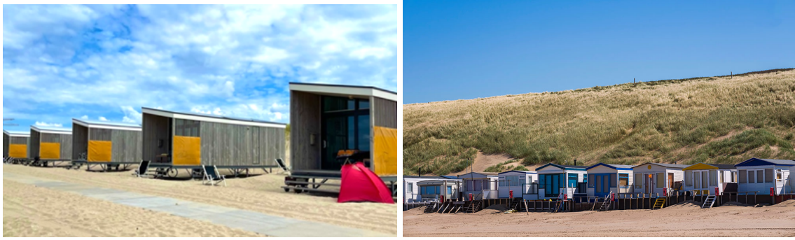
Figure 1: a. Beach buildings on the Zuiderstrand near Kijkduin, adopted from Pourteimouri et al. [1] and b. Beach buildings on the beach side of a coastal dune adopted from WOTY webpage on beach houses [2].
