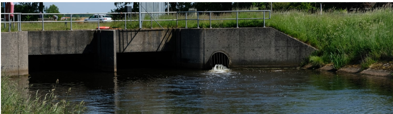
Figure 24: Discharge from the Almelo-De Haandrik canal to the Radewijkerbeek (Photograph taken by author on 28-5-2023)
