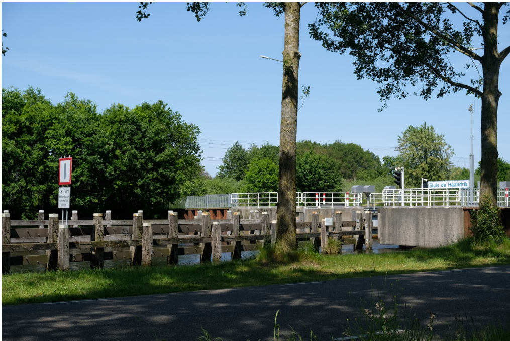
Figure 41: Photo: Entrance sluice de Haandrik
