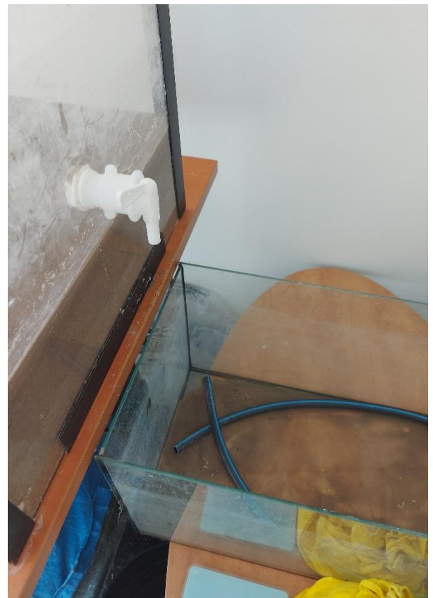
Figure 5.7: Water outlet with lower water tank
