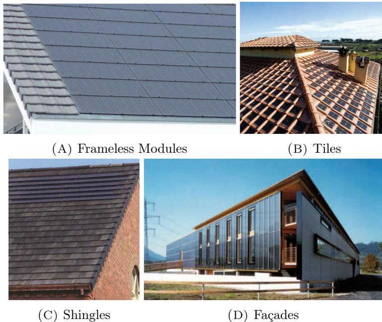
FIGURE 1.2: BIPV applied as A) frameless modules, B) tiles, C) shingles to roofs and D) to façades. Figures from [14]
