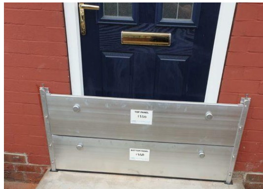
Figure 4 - Flood barrier in front of a door: a measure to minimize damage due to flooding (FloodSafe Projects, 2021)
