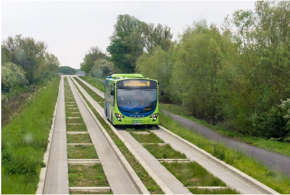
Figure 5: Cambridgeshire guided busway (Horgan, 2020)
