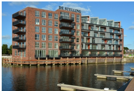
Figure 16, De Stelling building, a water robust construction (De Stelling, Zwolle, 2016)
