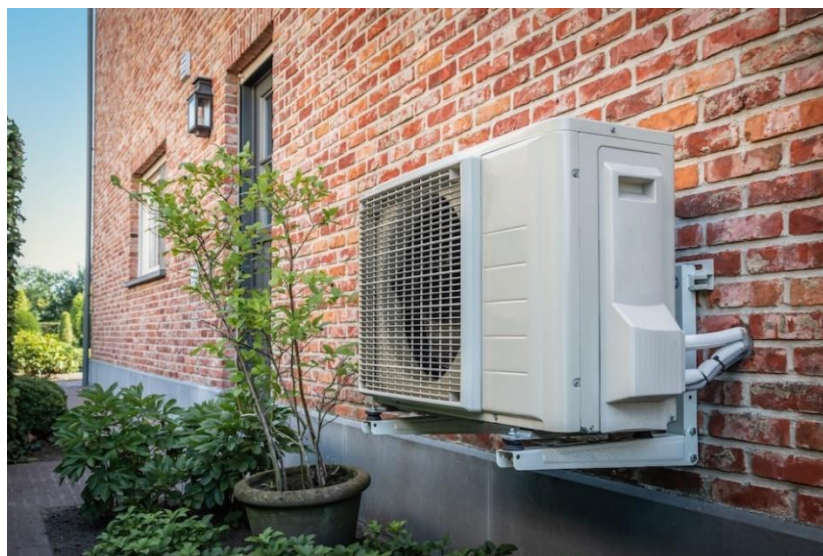
Figure 3: Outdoor unit of an electric heat pump
