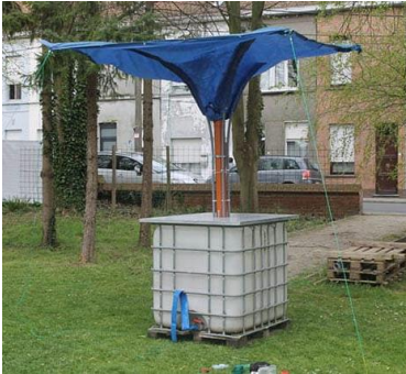
Figure 6: Stand-Alone Rainwater Collector [24].
